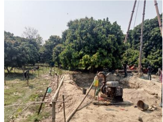
North - Eastern Side
