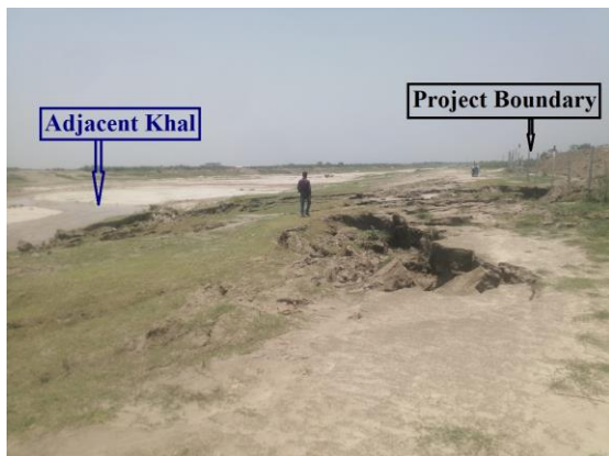
Adjacent Khal and Project Boundary
