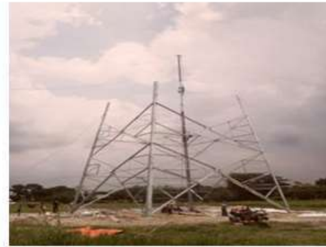
Tower erection work
