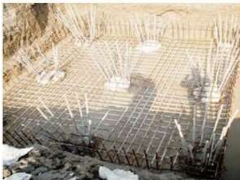
pile cap reinforcement
