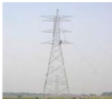
Tower erection works
