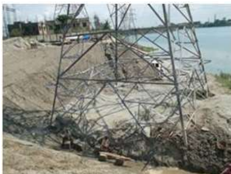
Placing tower on its foundation
