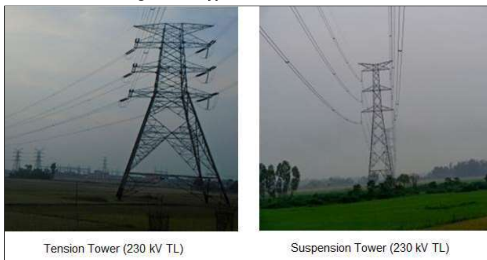
Figure 3.2: Type of transmission tower
