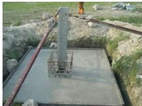
Casting CC into tower foundation
