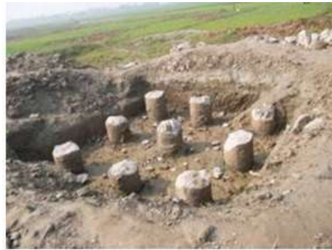
tower piling works
