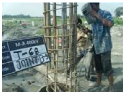
Welding of reinforcement
