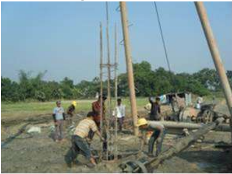
placing of steel ring bunds
