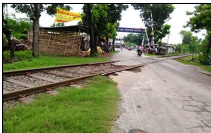
Figure 3.4: Railway crossing at Goalkhali Bus Stand
