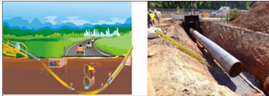
Figure 3.7: HDD process
