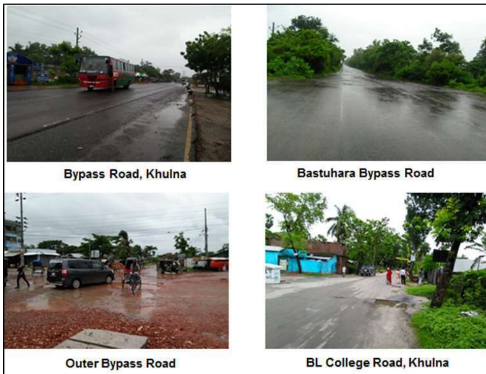
Figure 3.3: Some road crossings along the gas pipeline route
