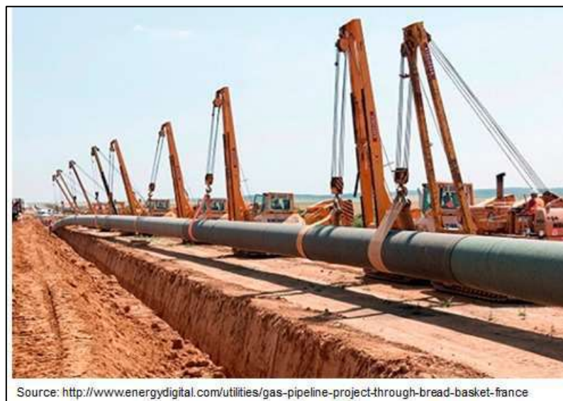
Figure 3.8: Laying of Pipeline
