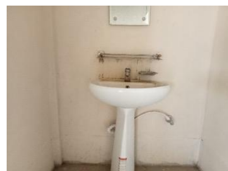
Wash Basin at The Dining Space
