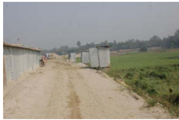
Single pit toilet facility
