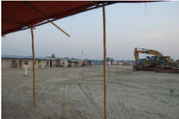
Site office and labour camp
