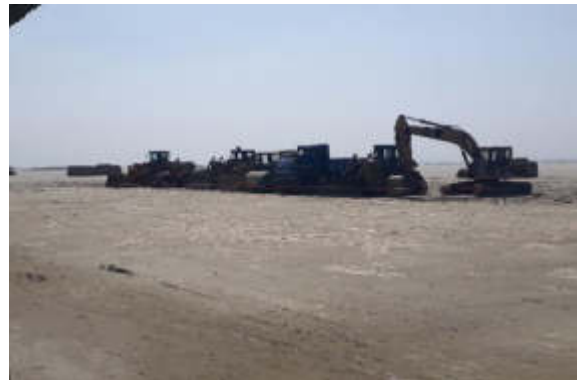
Construction machineries at site
