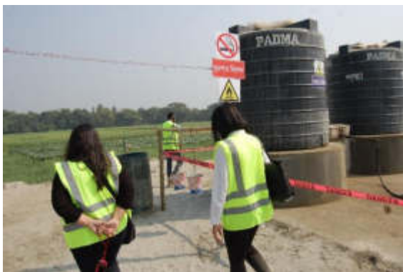
Diesel storage area with safety precaution
