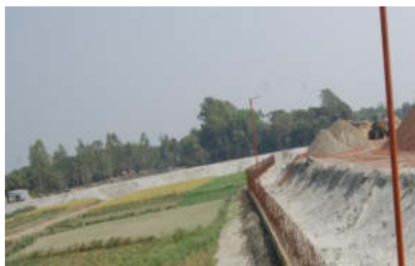
Site approach road
