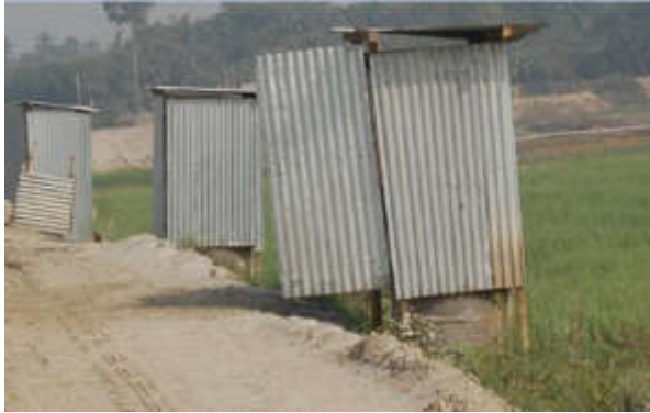
Single Pit Latrine
