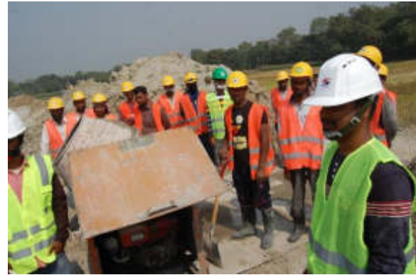
Workers with PPE at construction site
