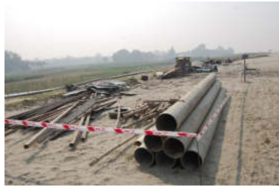
Construction junk material storage area
