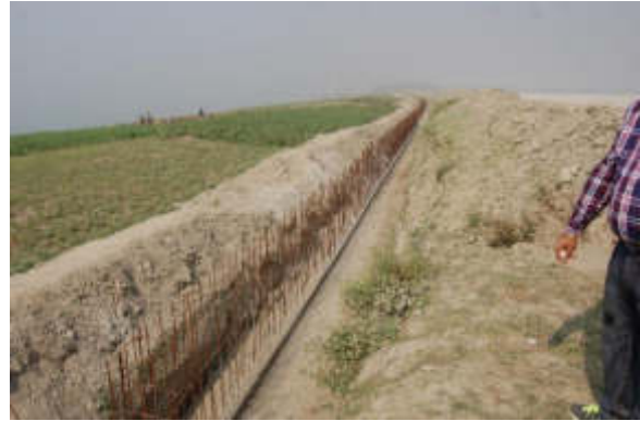
Construction of retaining wall (ongoing)
