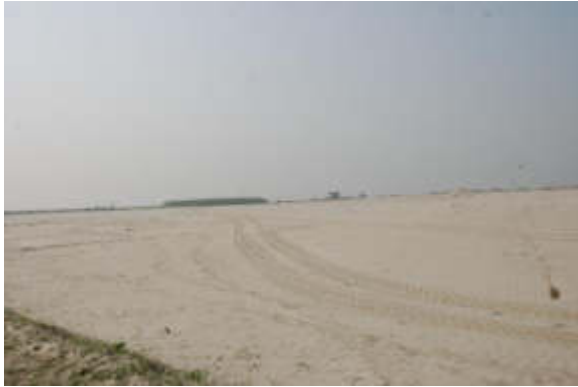
Site filled with Silver Sand
