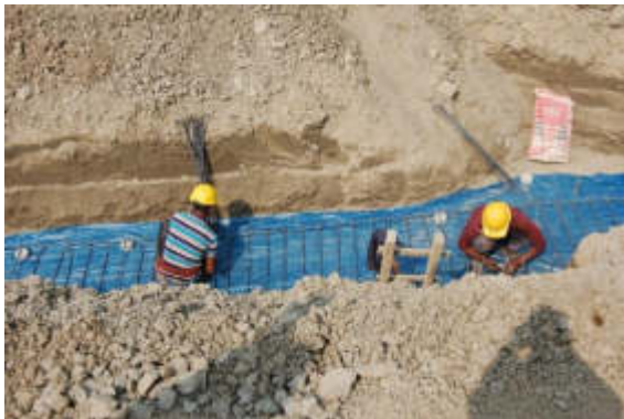
Construction of retaining wall (ongoing)
