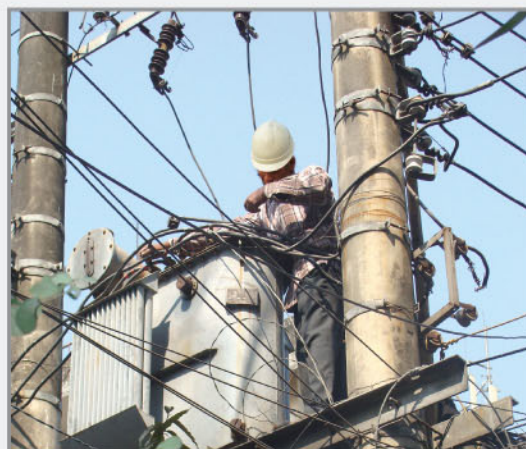
A BPDB Staff is in maintenance work of a Transformer
