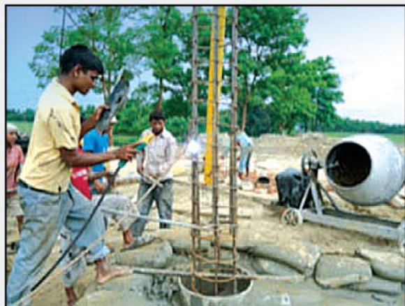
Rauzan 25 MW Power Plant Expected Commissioning Date : July 2012
