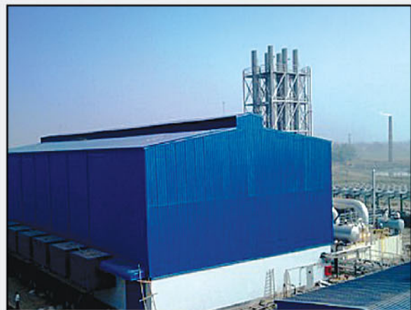
Gazipur 50 MW Power Plant Expected Commissioning Date : February 2012
